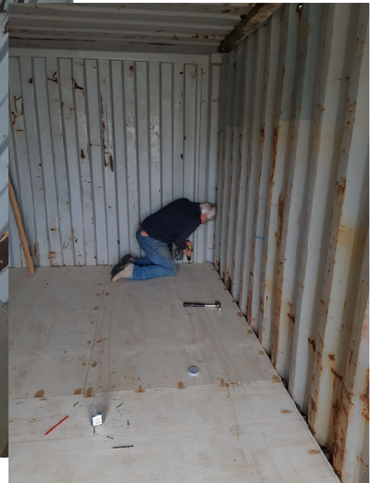
JG screwing down the last of new flooring
