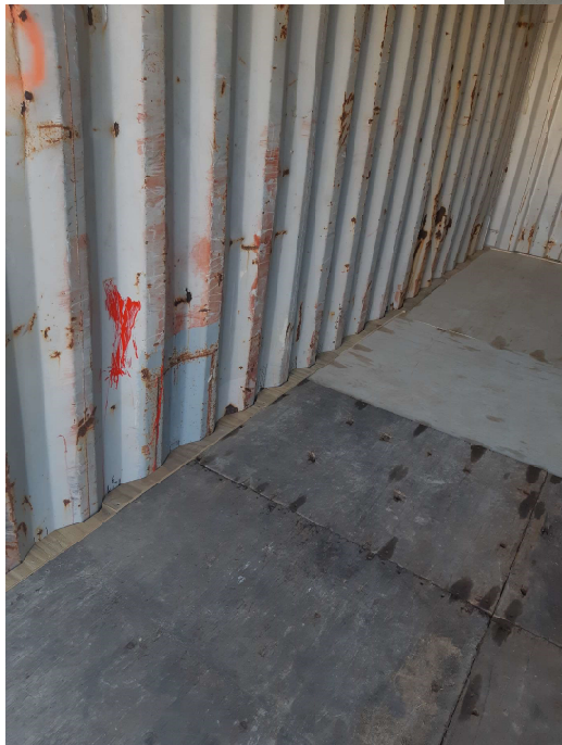
The old and new flooring with glimpse of joists
