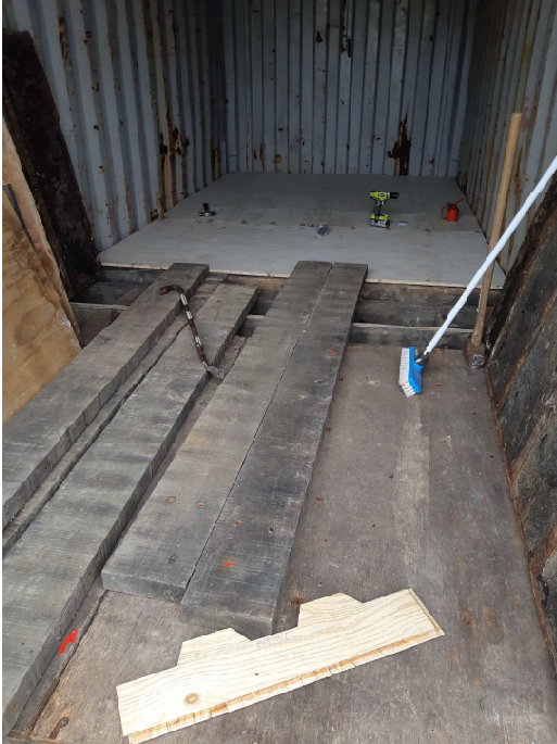
The old and new flooring with glimpse of joists
