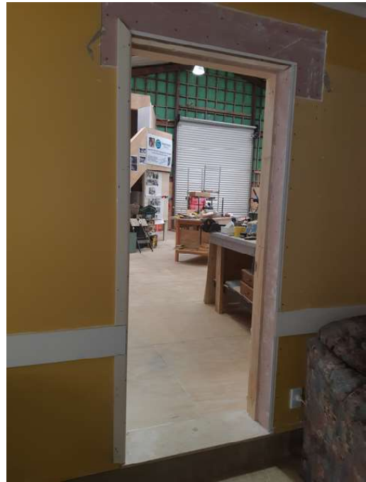
From kitchen side - just waiting for that architrave
