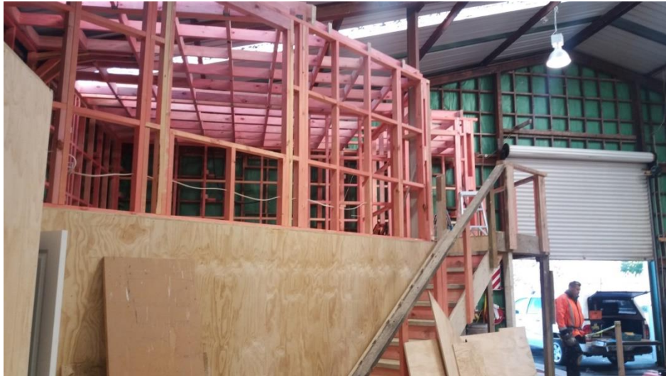
The mezzanine floor framed and ready for insulation and walls
